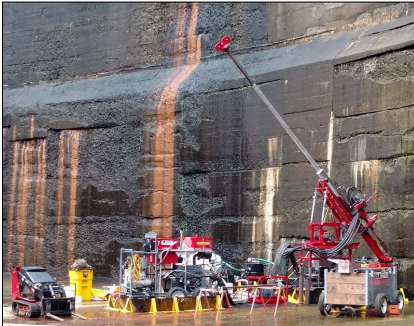
Figure 2. AAI diesel/hydraulic Ingetrol 75E drill rig at the toe of Walters Dam.
