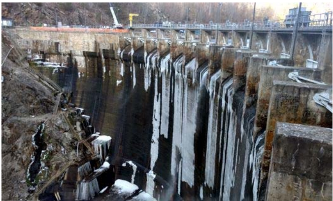
Figure 5. Accessing the drillholes using cranes.
