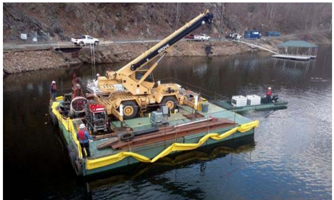
Figure 6. Access the drillholes using barges.
