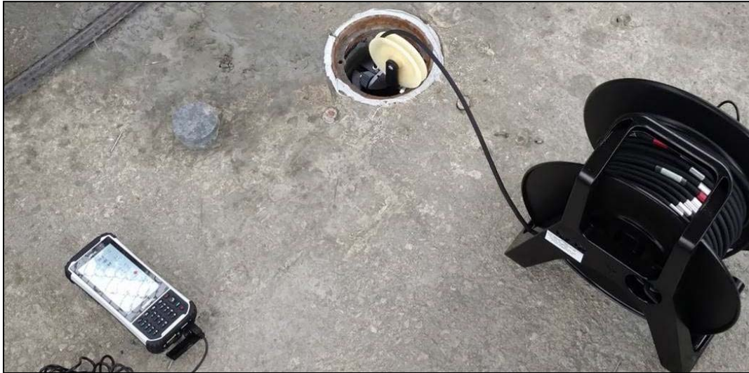
Figure 16. Hole OC-2 inclinometer baseline measurement recording.
