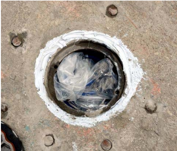
Figure 12. Hole OC-1 temperature probe and flush-mount cover photos.
